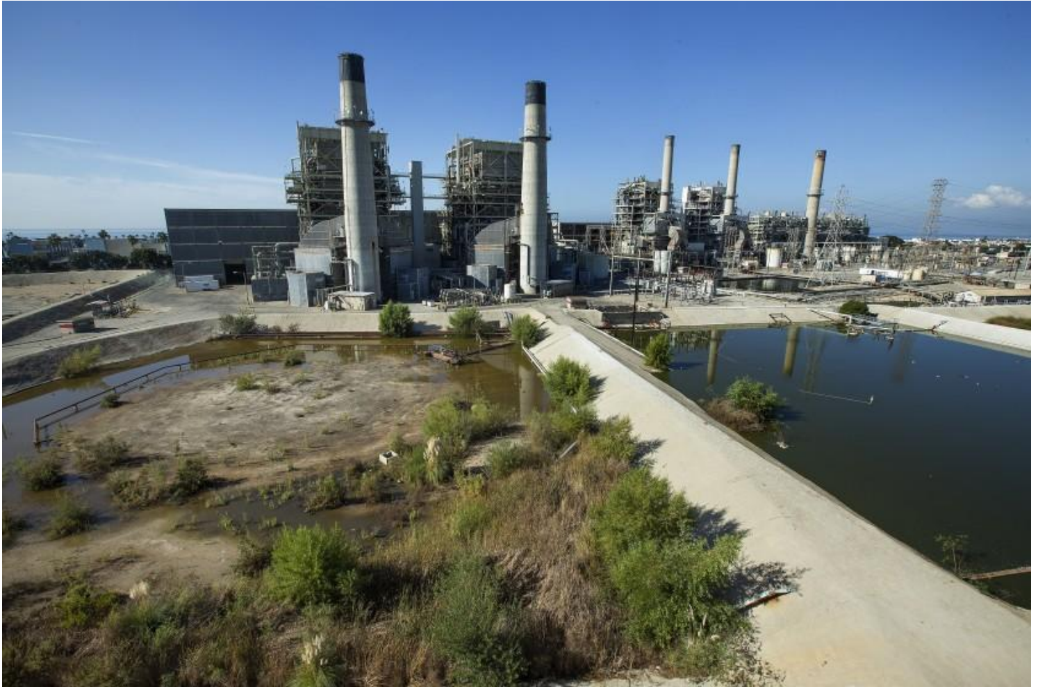
The gas-fired AES power plant in Redondo Beach. (Mel Melcon / Los Angeles Times)
